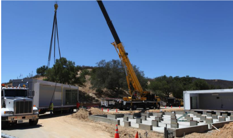
Figure 3. Oak Park High School site with GrowthPoint container readied by crane operator to place on foundation.
