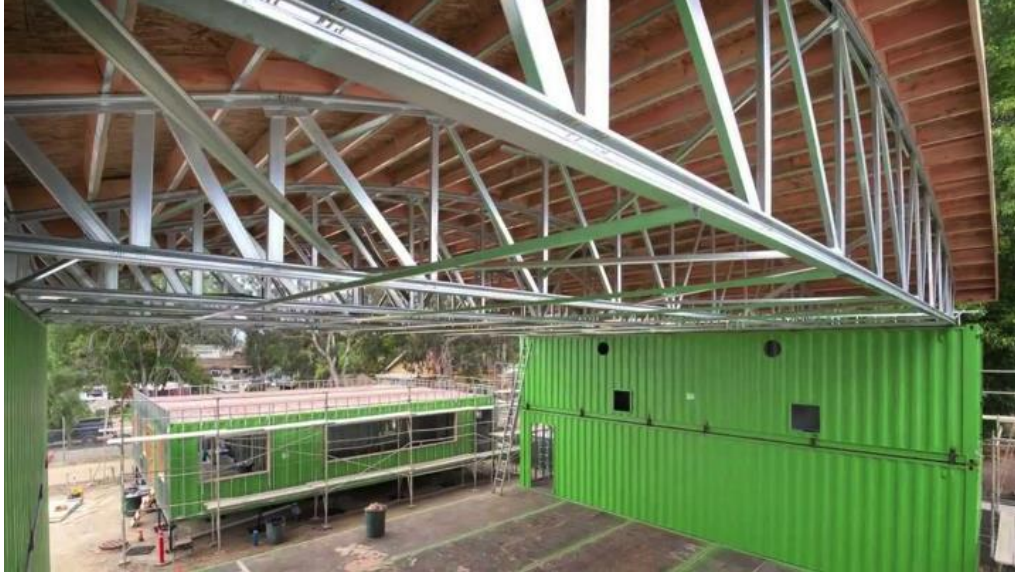
Figure 15. Waldorf School under construction from shipping containers in Costa Mesa, California.
