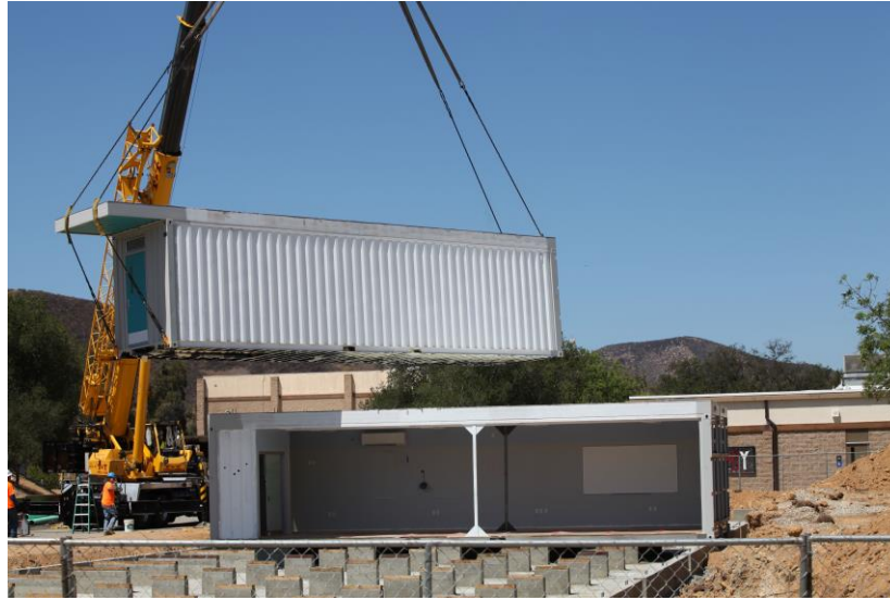
Figure 6. Twenty-one Growthpoint prefabricated containers were trucked in and placed on foundation at Oak Park High School site in one day.
