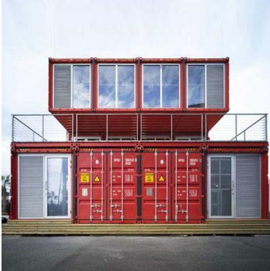
Figure 21. Puma City, 24 containers - transportable retail and event building that is traveling around the world. http://www.residentialshippingcontainerprimer.com/Puma%20Flexible%20Container%20Retail
